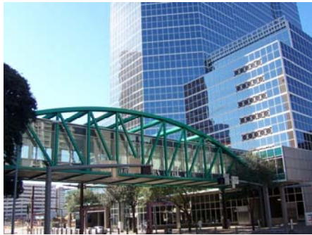
St. Luke's Episcopal Hospital – Fannin Street skywalk
