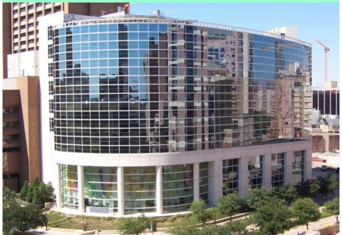
Texas Heart Institute — Denton A. Cooley Building
