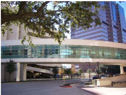
St. Luke's Episcopal Hospital – Garage No. 2 – skywalk
