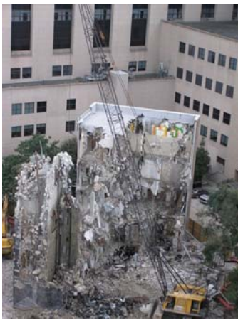
The Institute of Religion demolition
